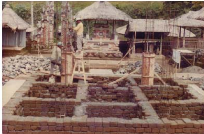
Restoration work in the temple, 1983
