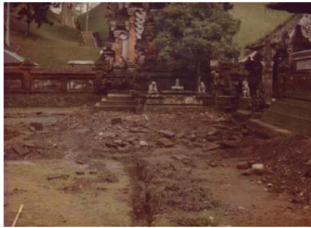
Condition of Tirta Empul after earthquake disaster, 1972
