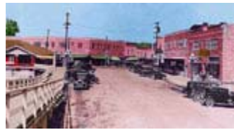
▣ Figure 2 Looking east from the Ferry Dock, circa 1920s
