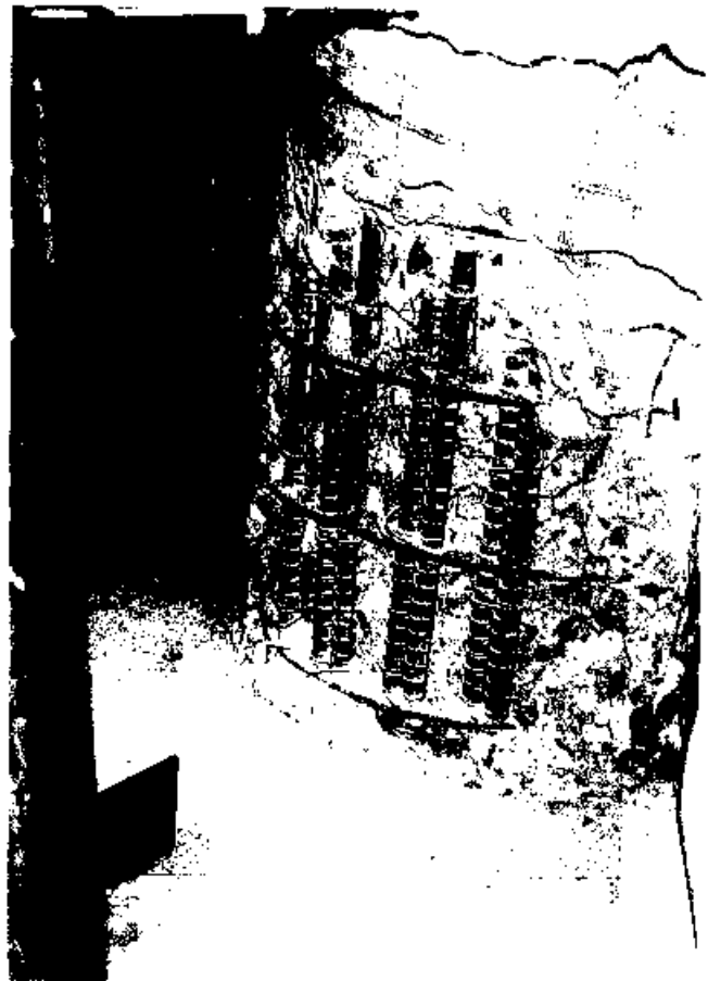
Fig. 22—Bond failure of Column C-1
