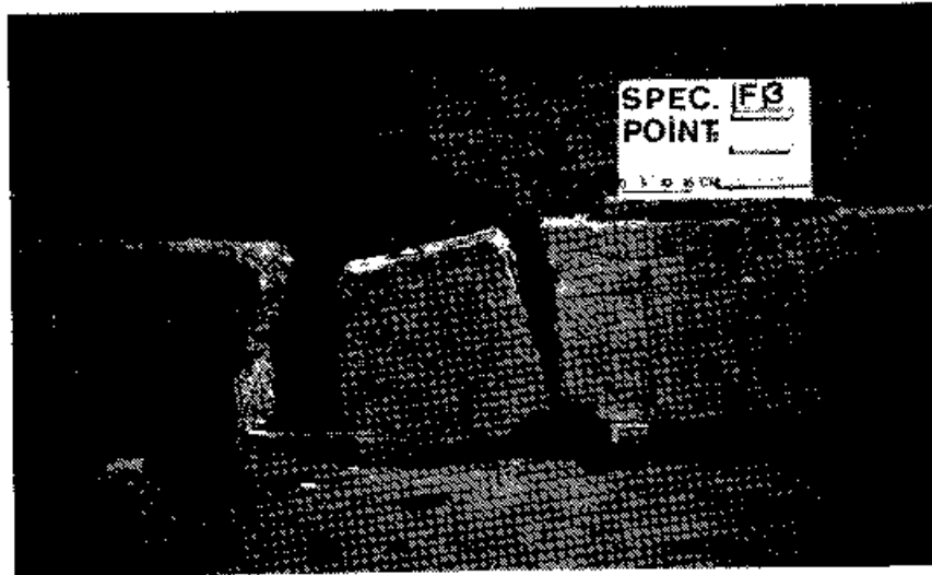
Figure 9. Beam F3 at failure.
