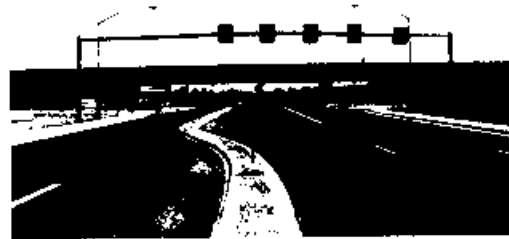
FIG. 2.—100-ft Monotube Structure Located in Phoenix, Arizona
