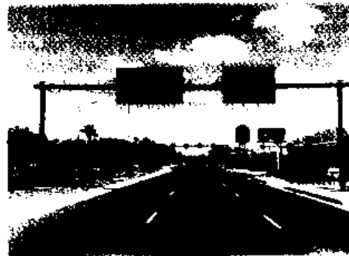
FIG. 1.—60-ft Monotube Structure Located in Tucson, Arizona
